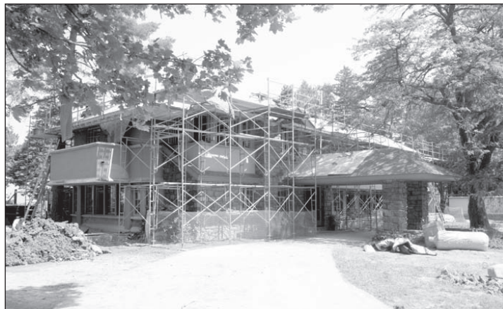
Graycliff under restoration - 2006
