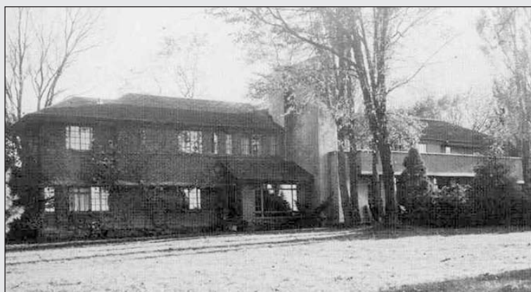
A 1950's card of Graycliff lakeside, published by the Piarist Fathers , showing the chimney prior to stone restoration
